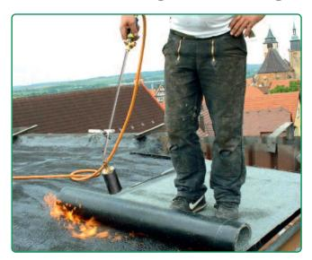
The PERKEO TITAN is a featherweight roofing + heating torch, whose component parts have been constructed from that extraordinary metal - titanium.
